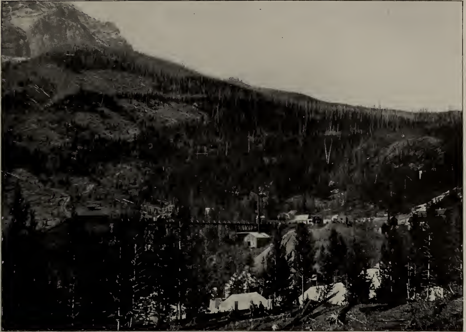
TIPPLE AND ENTRANCE TO MINE, BANKHEAD, ALBERTA.
